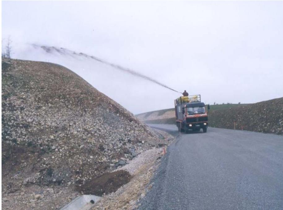
**Figure 2. Hydroseeding technique particularly adapted to revegetate steep slopes and hard access areas.**
