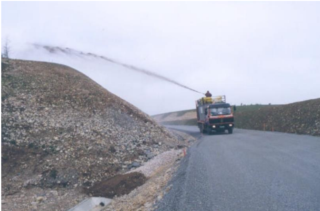
Figure 1. Utilizing hydroseeding technique as a restoration tool on a steep road cut slope.
